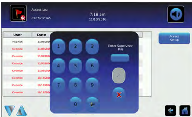
Access Control Setup screen with password keypad overlay
