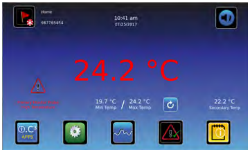
Home screen with active alarm
