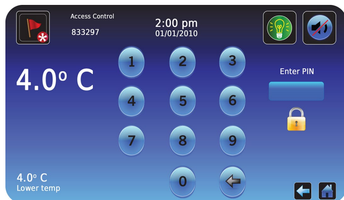
Access Control keypad
