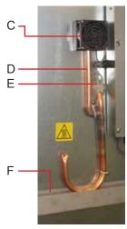
Left: Unit cooler (A) inside the chamber, with drain port (B). Right: drain line fan (C), drain tubing (D), and heater wires (E).
