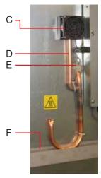
Left: Unit cooler (A) inside the chamber, with drain port (B). Right: drain line fan (C), drain tubing (D), and heater wires (E).
