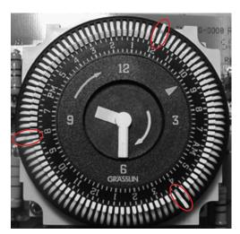
Horizon Series defrost controller with defrost times set to On position at 12:00 AM, 8:00 AM, and 4:00 PM.
