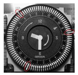
Defrost controller with defrost times set to On position at 12:00 AM, 8:00 AM, and 4:00 PM.
