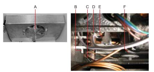
Left: Unit cooler. Right: Unit cooler interior.
