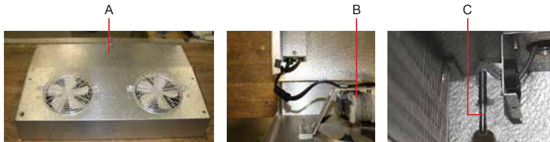
Left: Unit cooler. Center and right: Unit cooler parts.
