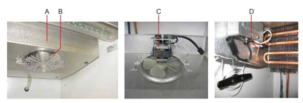
Left: Unit cooler with fan guard. Middle: Unit cooler fan. Right: Temperature control probe.
