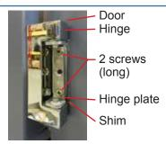
Attach hinge to door (lower hinge shown).
