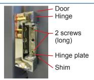
Attach hinge to door (lower hinge shown).
